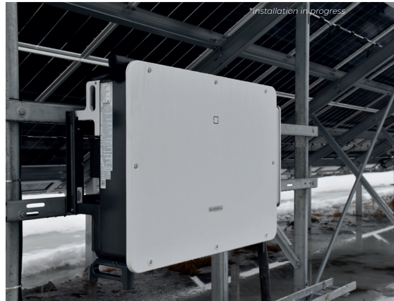
Inverters are installed under the PV module structure. Enclosure surface is frozen but doesn't affect functionality.
